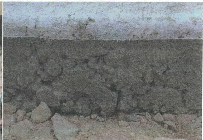
Consolidate concrete along the form edges to avoid honeycombing.
