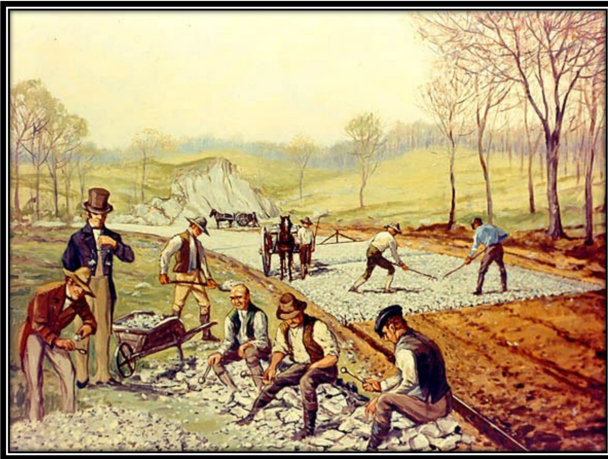
Construction of a macadamized road ca. 1823
