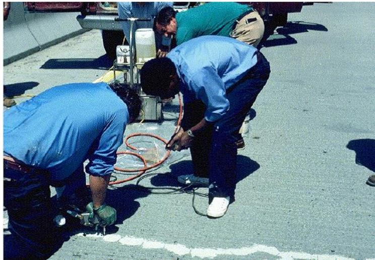
**Figure 31. Epoxy Injection Procedure (VirginiaDOT 2009)**
