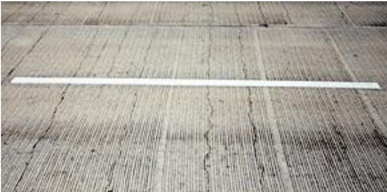
**Figure 1. Early-age shrinkage cracking of a bridge deck (Kosmatka and Wilson 2011)**
